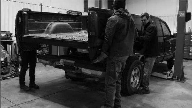
Hold the part up to the frame and mark off its coverage. Use the frame holes and angles to align it correctly.
