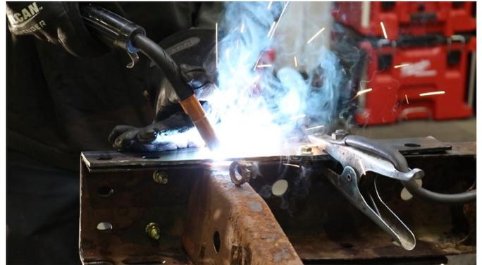
Make sure to weld completely around all edges to prevent future rust and corrosion to the frame rail.
