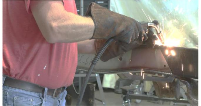
To ensure a tight fit, screw the two bolts on the end in with a 15mm socket before welding the rest of the frame section into place.
