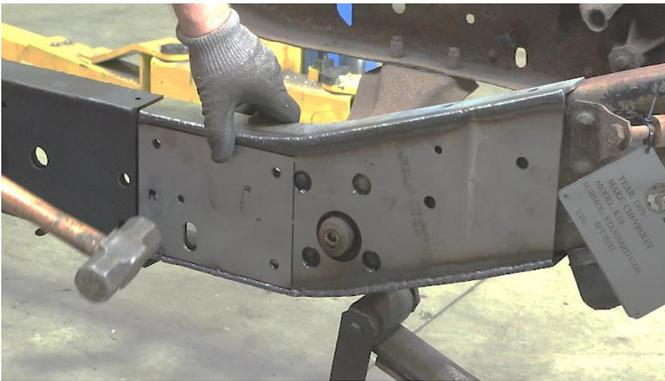
With a 15mm socket and 14mm wrench, screw in the bolts and nuts, holding the front cab mount in place.
