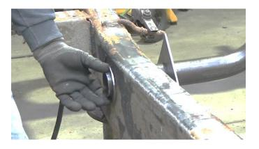
Following proper welding procedures, tac weld your driveshaft crossmember onto the frame before welding it on fully. Weld 100% around all edges.
