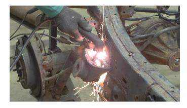
Grind down the frame free of rust and debris, revealing bare metal.
