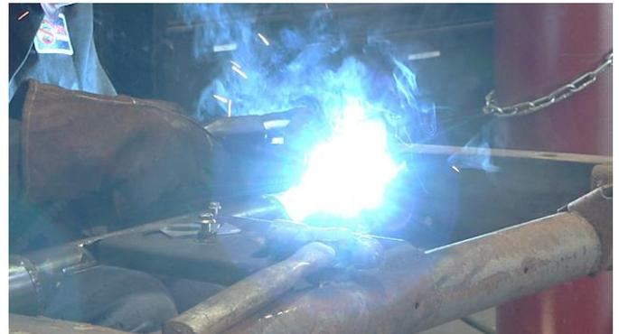
Once in place, finish welding around the support plates followed by welding your crossmember into place. Weld 100% around all edges.
