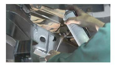
Following proper welding procedures, tac weld the part onto the frame before welding it on fully. Weld 100% around all edges.
