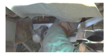
Once in place, finish tac welding the part onto the frame before welding the part on fully. Weld 100% around all edges.
