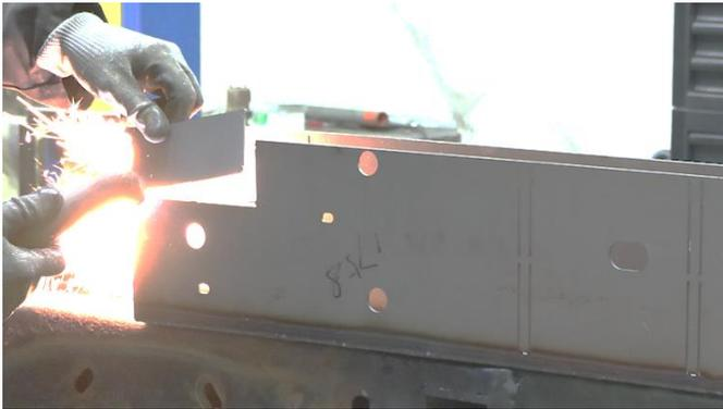
Our part also features a perforated plate you can remove to fit over your existing center cab mount. If you decide to keep your cab mount, cut out the perforated plate. If not, remove your cab mount.
